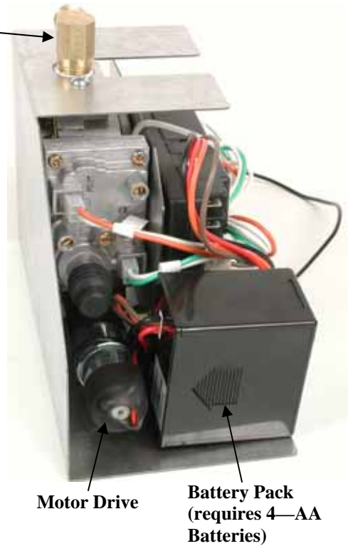
Figure 4—Front of Control Assembly
